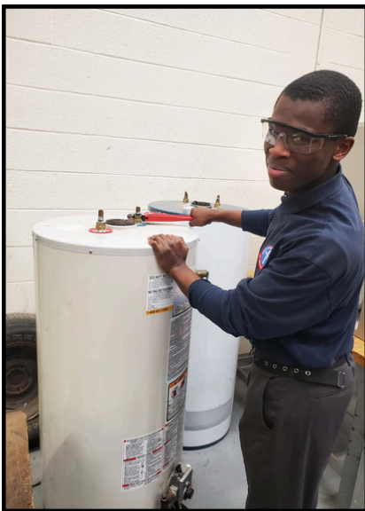
Godswill installing a brass fitting on a hot water tank
